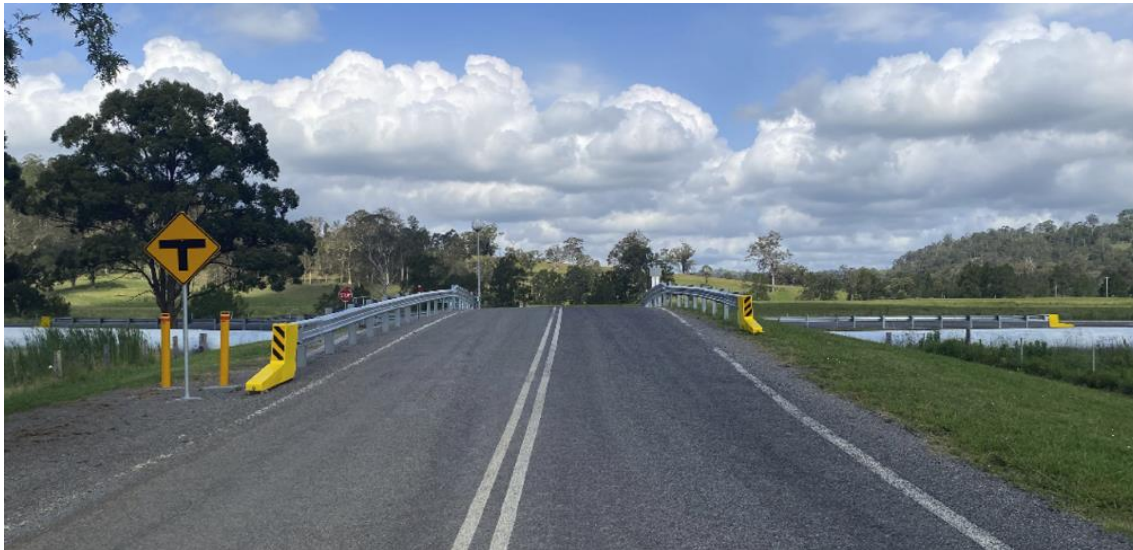
Figure 3.5: Hanleys Creek Road Facing West Towards Clarence Town Road (November 2024)
